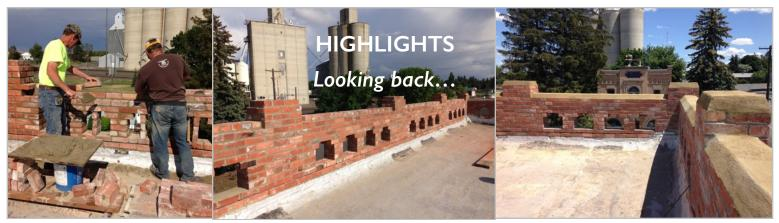
June 2015 -Blayne Foley and his crew rebuilt the Hotel Lincoln parapet walls. The picture on the upper right is the finished "topped" brick. Foley carefully rebuilt each chimney that were originally used for the coal stoves that heated each hotel room.
